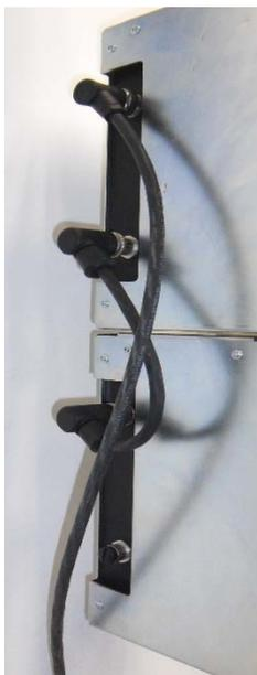
Now the individual luminaires are connected with the LEDSecure SOL interconnecting cable. As well as the first lighting module connected with the secondary-side connection cable which is then also connected to the mains unit. The unused plugs on the luminaires must be locked via the blank cover.
